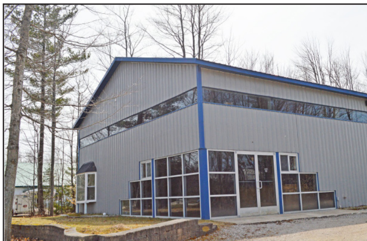
8580 Commerce Court, Harbor Springs.
